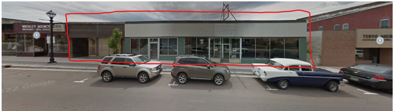
^Street view of the building to be demolished.
